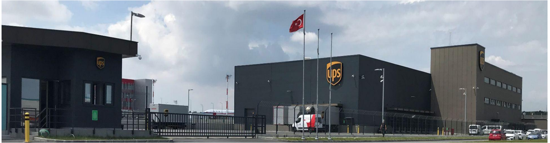
UPS Gateway Center in Istanbul, Türkiye, 12.000 m 2
